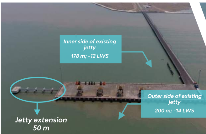
Extension of Multipurpose Jetty 250m x 50m in progress
